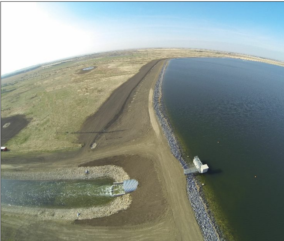
The Langdon Reservoir capacity was doubled last winter to 12000 acre/feet. This provides increased drought insurance for the District.
