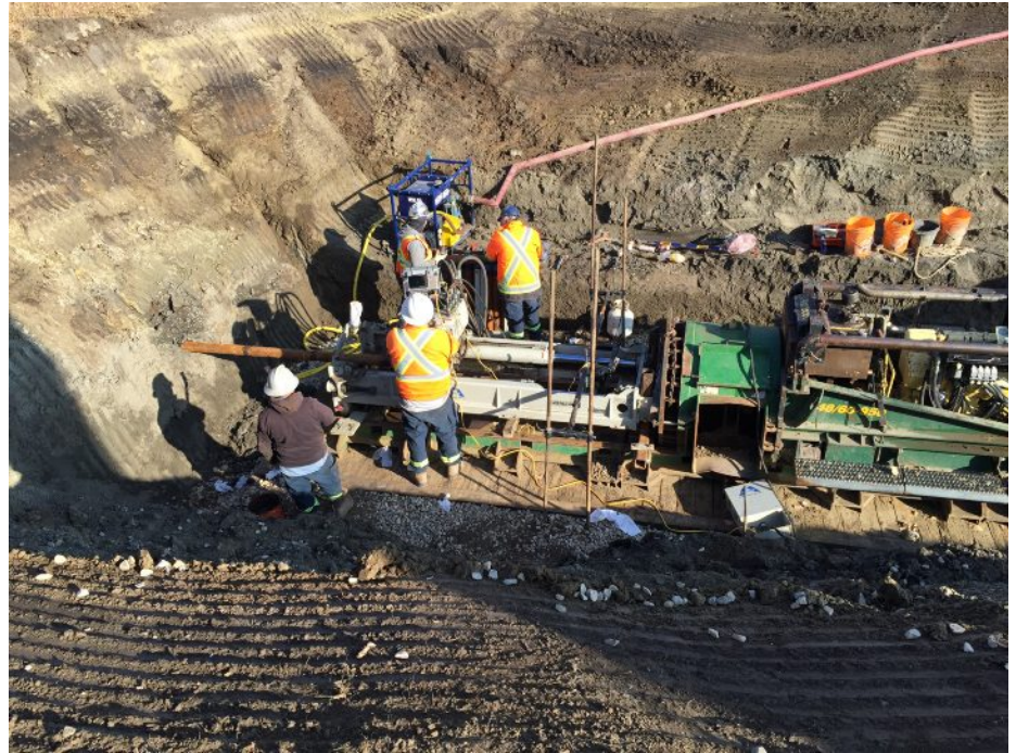
WID crews bore under Highway 561 to install pipeline - WID photo
