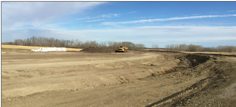
C Canal undergoing preparation for liner installation - WID photo
