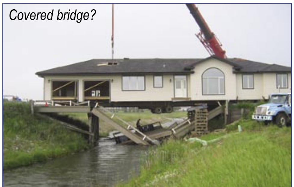
Here’s an example of an unexpected Operations Department emergency that took place last season. Not quite your average covered bridge. Photo by Erwin Braun
