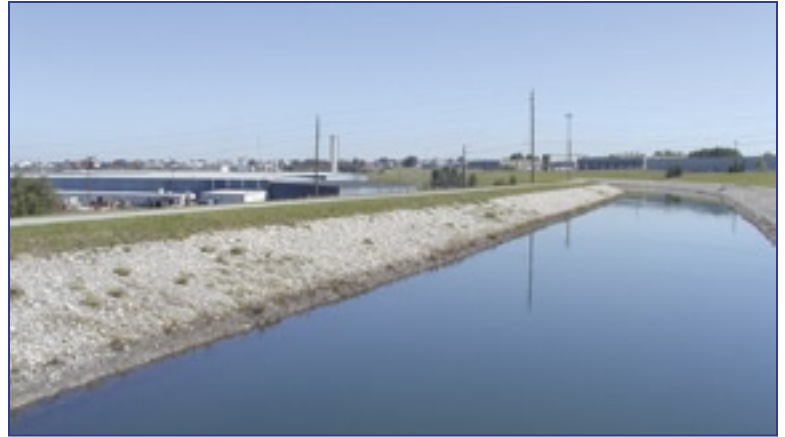
Western Headworks canal as it travels through industrial Calgary Photo: C. Lacombe
