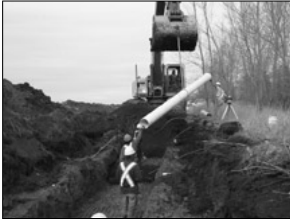
Grove pipeline going into the ground. WID photo
