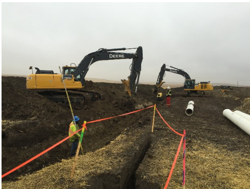
Pipeline installation near Standard - WID photo
